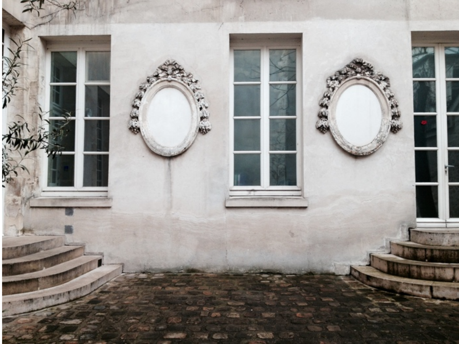
Folly No. 3: Empty frames in a courtyard off Rue de Turenne
