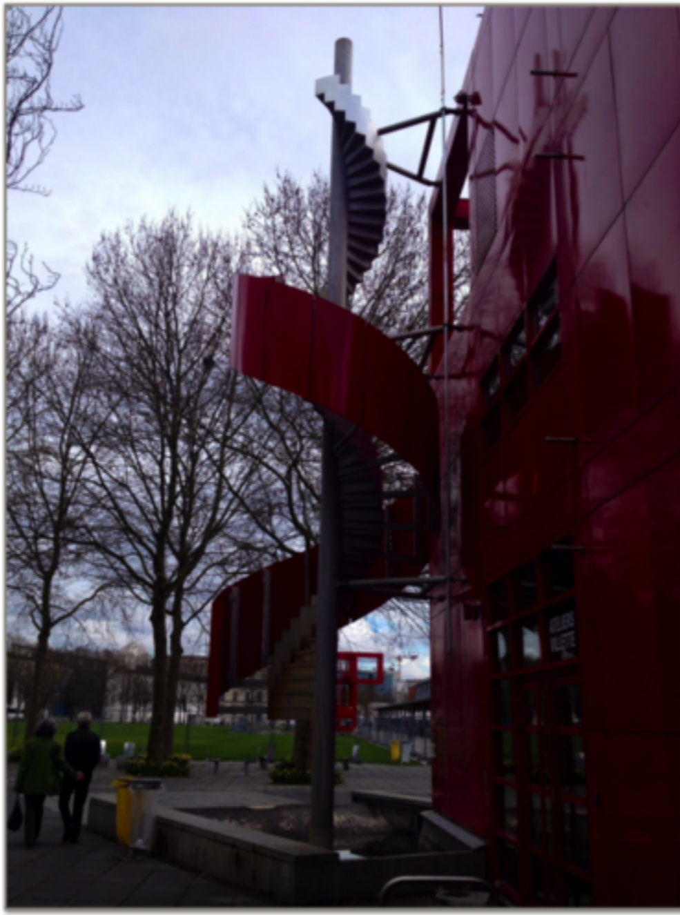
Folly No. 1: One of architect Bernard Tschumi's 35 follies in Parc de la Villette
